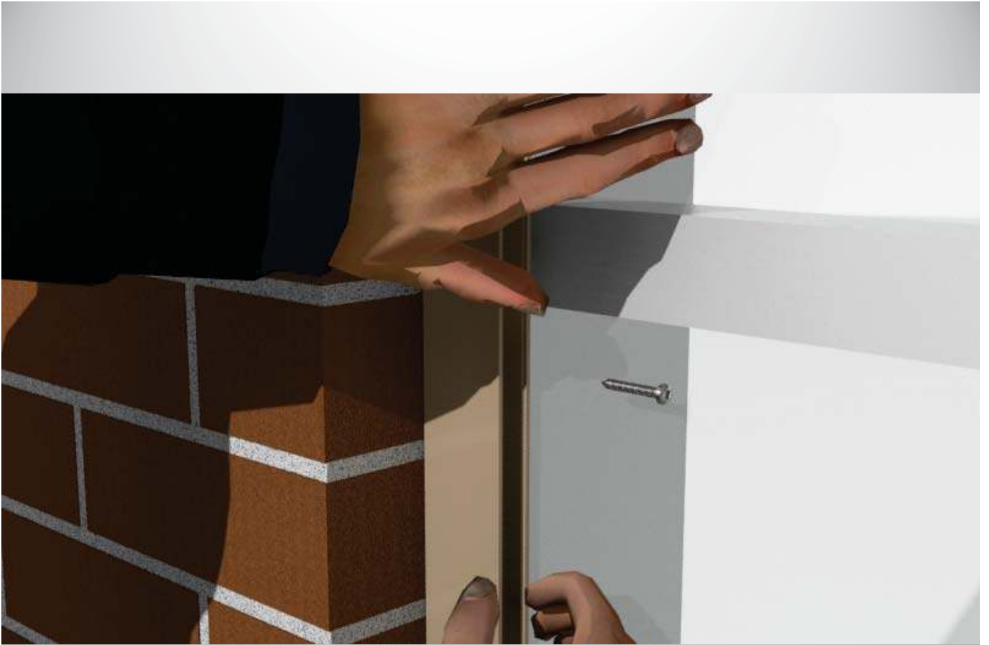
Step 23: Secure the shutter guides using the provided screws.
