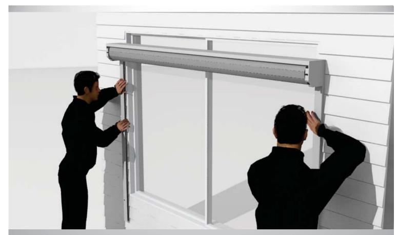
Step 21: For lifting the shutter, two people will need to hold the assembly on both sides and lift at the same time to place it on the wall. Then slide it up in place while pushing against the wall.
