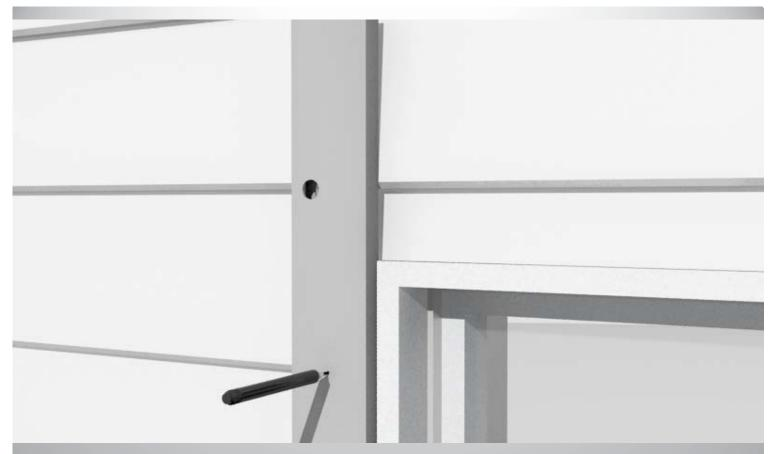
Step 5: Mark at least 3 fixing points on the packer approx. 100 mm from the top and bottom and distribute the holes approx. 400~500 mm apart making sure you place the holes over the bullnose (the highest point on the timber).
