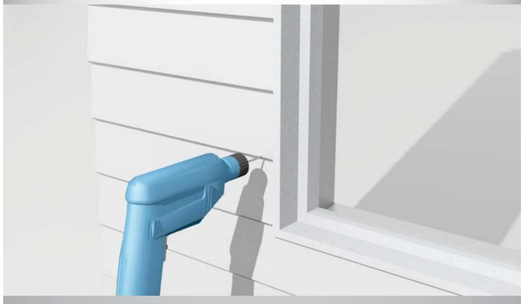
Step 12: Use the 3 mm drill bit to drill pilot holes for securing points including the pelmet box fixing point.
