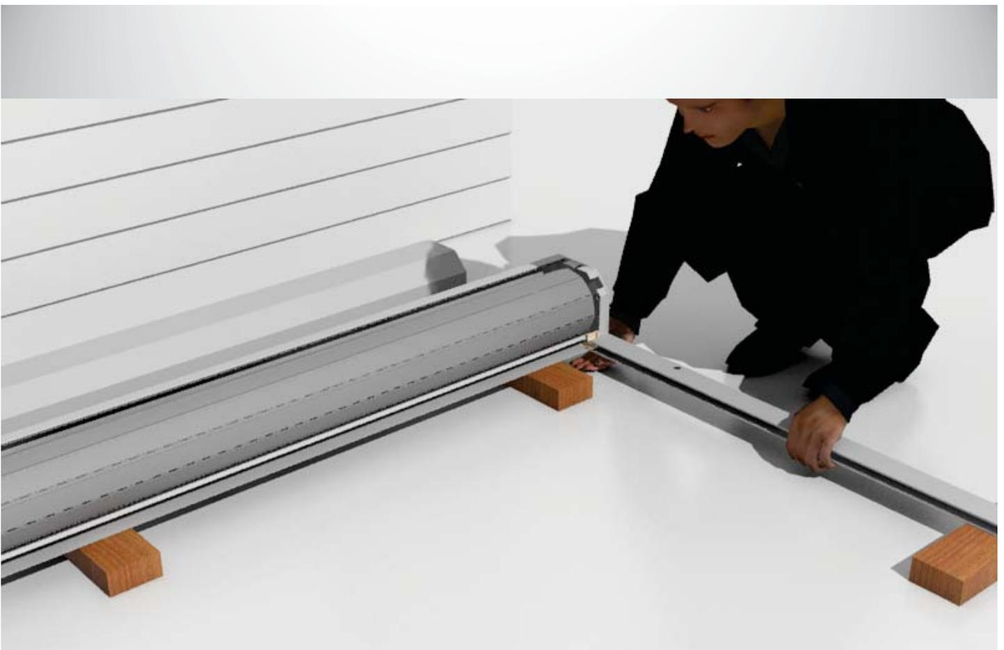
Step 20: Shutter is now ready to be secured on the wall. Put one hand underneath the pelmet box and the other holding the shutter guide. Avoid tilting the guides as this may break the legs.
