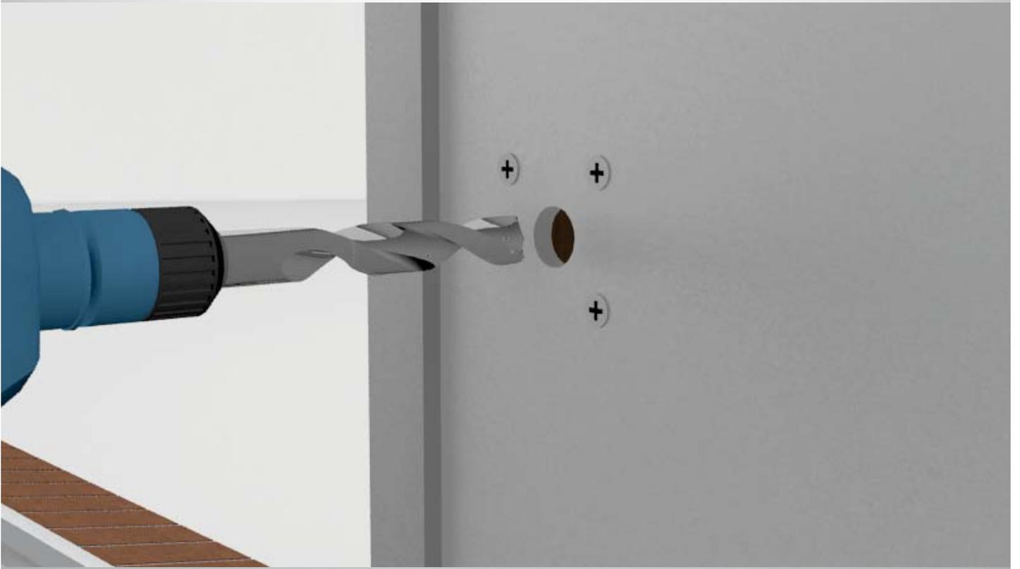
Step 27: Drill a hole in the centre for the cable.
