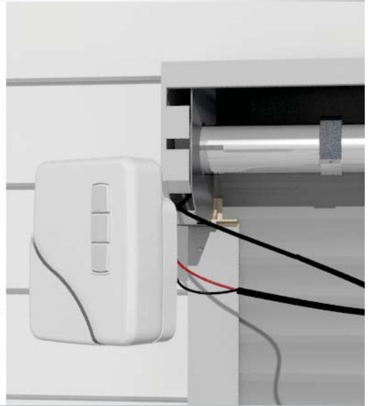
Step 23: Before wiring the DC motor, the roller shutter must be closed to have access to feed the cable into the wall cavity. Connect the motor temporarily by using the battery handset and handset holder to operate and close the roller shutter. [Note: Make sure your battery handset is charged]
