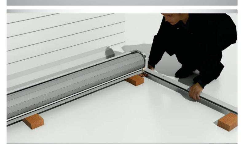
Step 20: Shutter is now ready to be secured on the wall. Put one hand underneath the pelmet box and the other holding the shutter guide. Avoid tilting the guides as this may break the legs.
