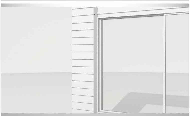
Step 4: Place one of the packers on the wall, keeping it flush with the bottom of the opening.
