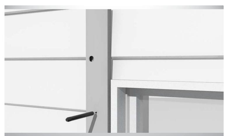
Step 5: Mark at least 3 fixing points on the packer approx. 100 mm from the top and bottom and distribute the holes approx.  $400^{\circ}500$  mm apart making sure you place the holes over the bullnose (the highest point on the timber).
