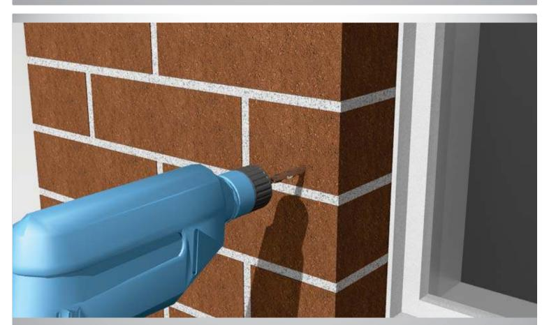
Step 12: Use the 6.5 mm masonry drill bit to drill holes at 35 mm depth on the wall for all fixing points including the pelmet box fixing point.
