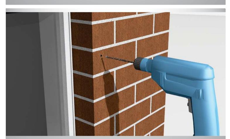
Step 18: Use the 6.5 mm masonry drill bit to drill holes at 35 mm depth on the wall for all fixing points including the pelmet box fixing point.
