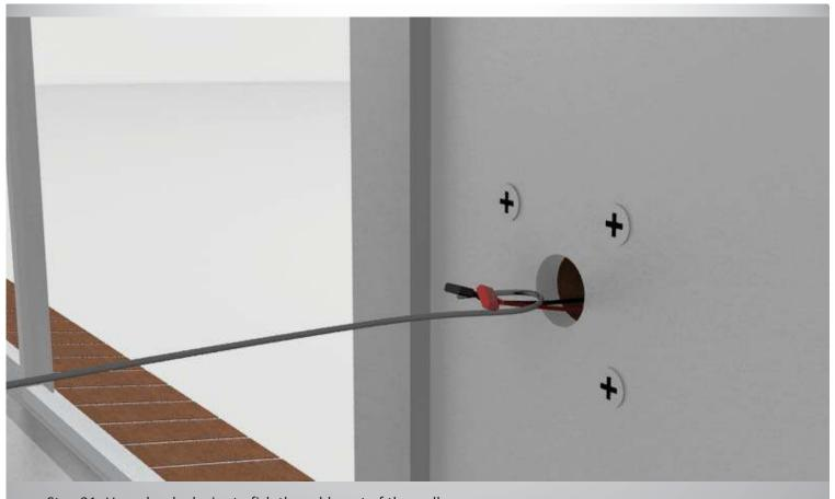
Step 31: Use a hooked wire to fish the cable out of the wall.
