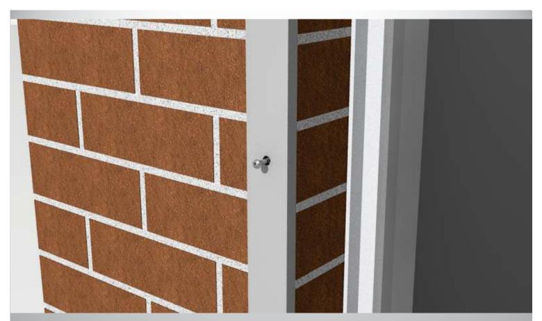
Step 15: Secure the packer on the wall using the provided screws.
