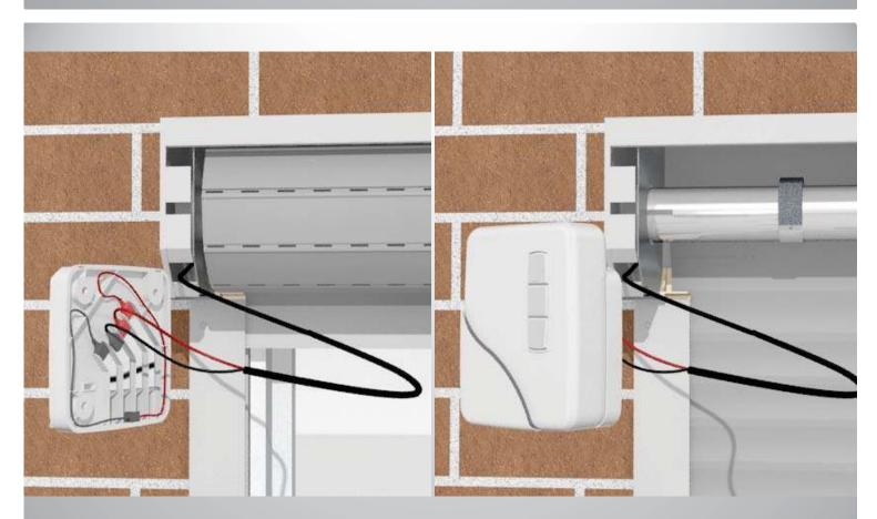
Step 26: Before wiring the DC motor, the roller shutter must be closed to have access to feed the cable into the wall cavity. Connect the motor temporarily by using the battery handset and handset holder to operate and close the roller shutter.
