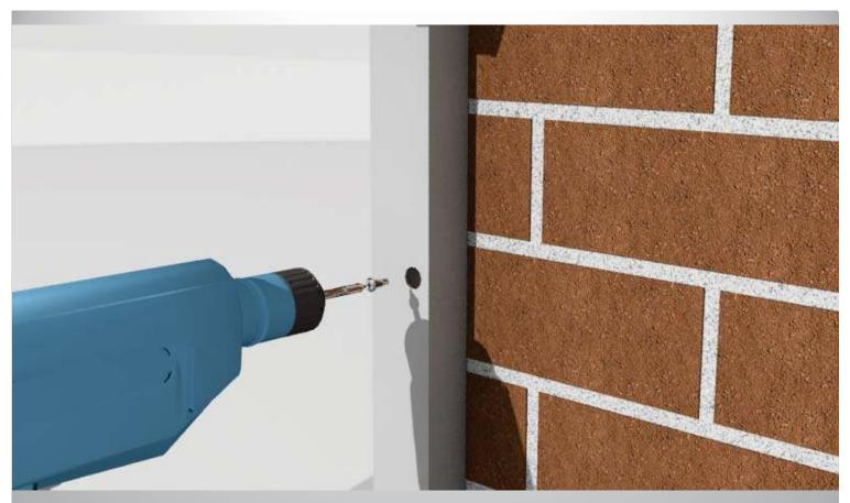
Step 25: Use the provided TEK screws and a drill-driver to secure the shutter guides on the packers. After putting all the screws in, use the plastic caps to cover the holes.
