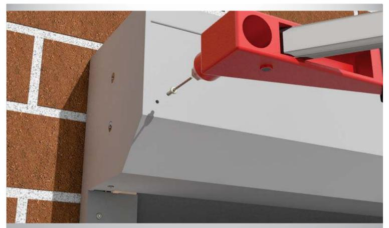
Step 35: Put the front cover in place by sliding it in and securing it using the provided rivets into the pre-drilled holes.
