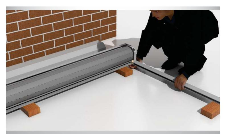
Step 23: Shutter is now ready to be secured on the wall. Put one hand underneath the pelmet box and the other holding the shutter guide. Avoid tilting the guides as this may break the legs.
