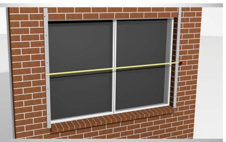
Step 16: Put the other packer on the wall and space it so that the overall measurement of the packers is the same as the overall width of the pelmet box. Measure the top and bottom distance to make sure the packers are parallel.
