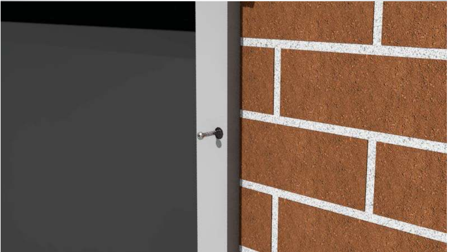
23. Secure the guides using the provided screws.
