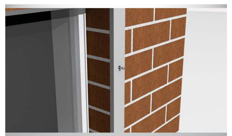
Step 19: Secure the packer on the wall using the provided screws.
