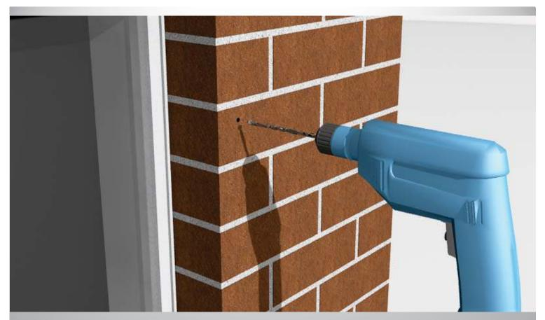
Step 17: Use the 6.5 mm masonry drill bit to drill holes at 35 mm depth on the wall for all fixing points including the pelmet box fixing point.
