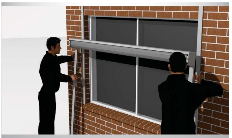
Step 23: For lifting the shutter, two people will need to hold the assembly on both sides and lift at the same time to place it on the wall. Then slide it up in place while pushing against the wall.
