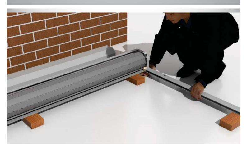
Step 22: Shutter is now ready to be secured on the wall. Put one hand underneath the pelmet box and the other holding the shutter guide. Avoid tilting the guides as this may break the legs.
