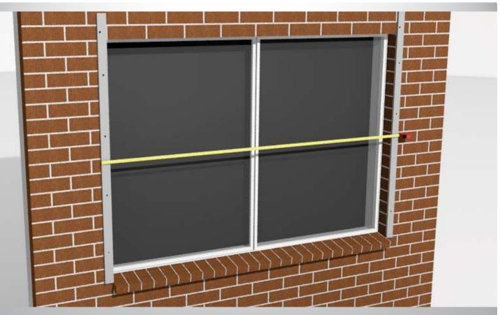
Step 15: Put the other packer on the wall and space it so that the overall measurement of the packers is the same as the overall width of the pelmet box. Measure the top and bottom distance to make sure the packers are parallel.
